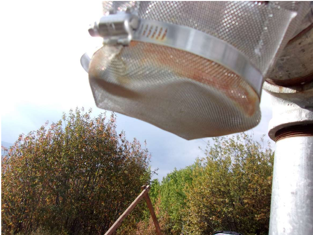
Roof Vent Screen
