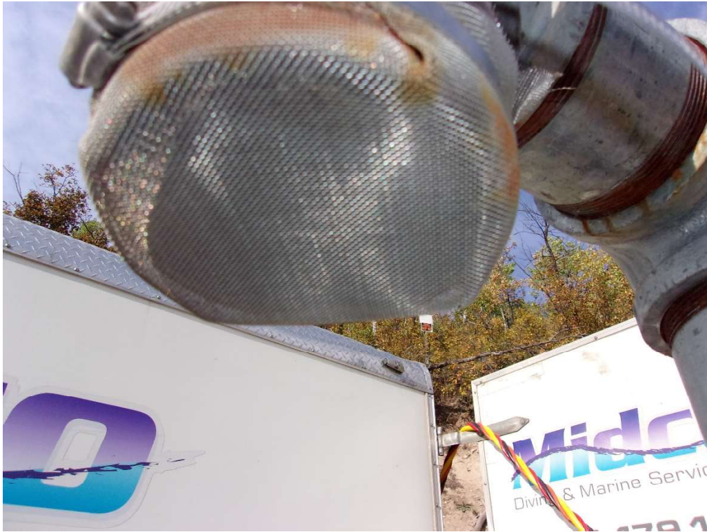
Roof Vent Screen
