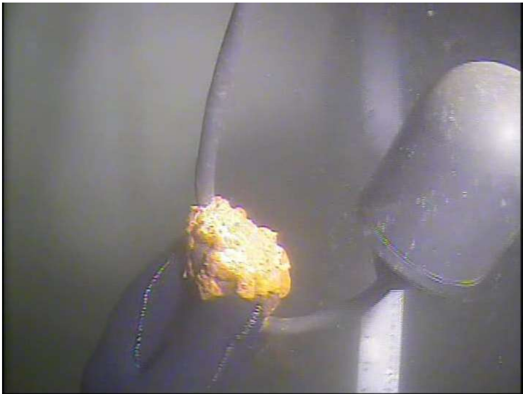
Telemetry Sensor – Corrosion Noted
