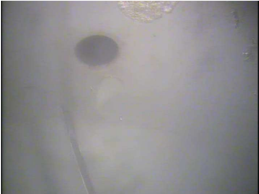
Interior Roof Vent
