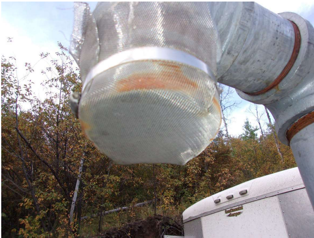
Roof Vent Screen
