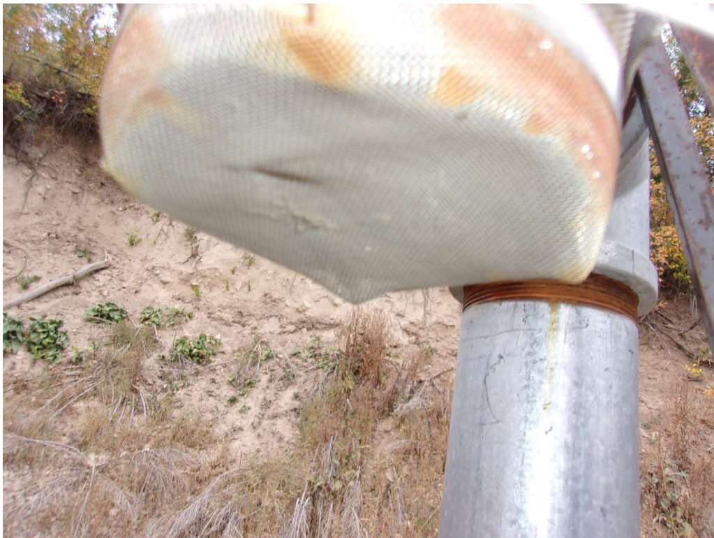
Roof Vent Screen
