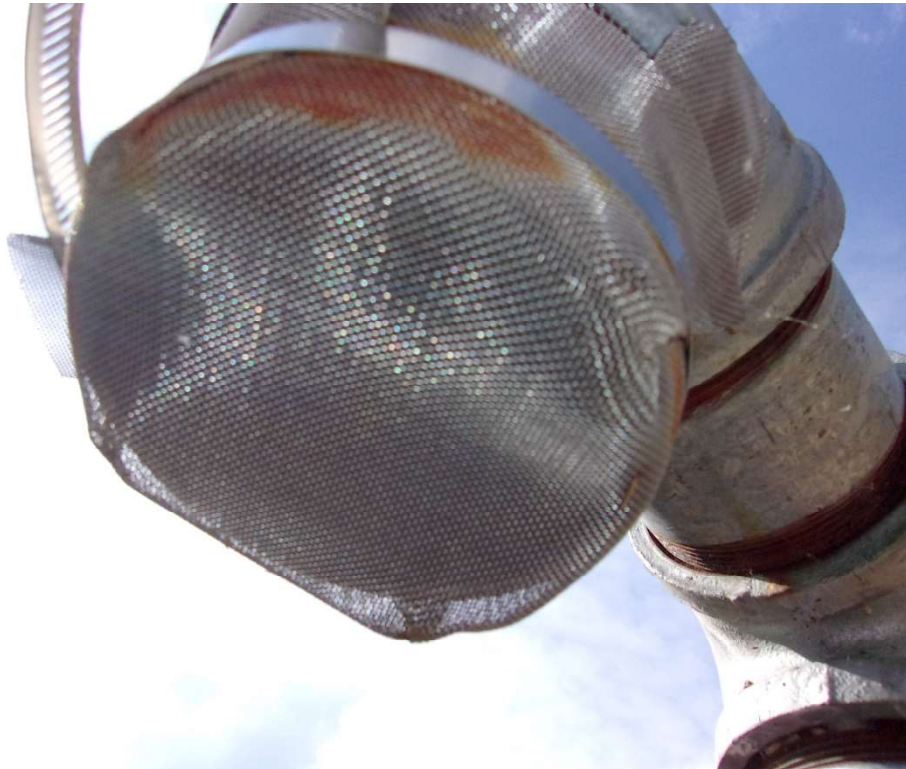
Roof Vent Screen
