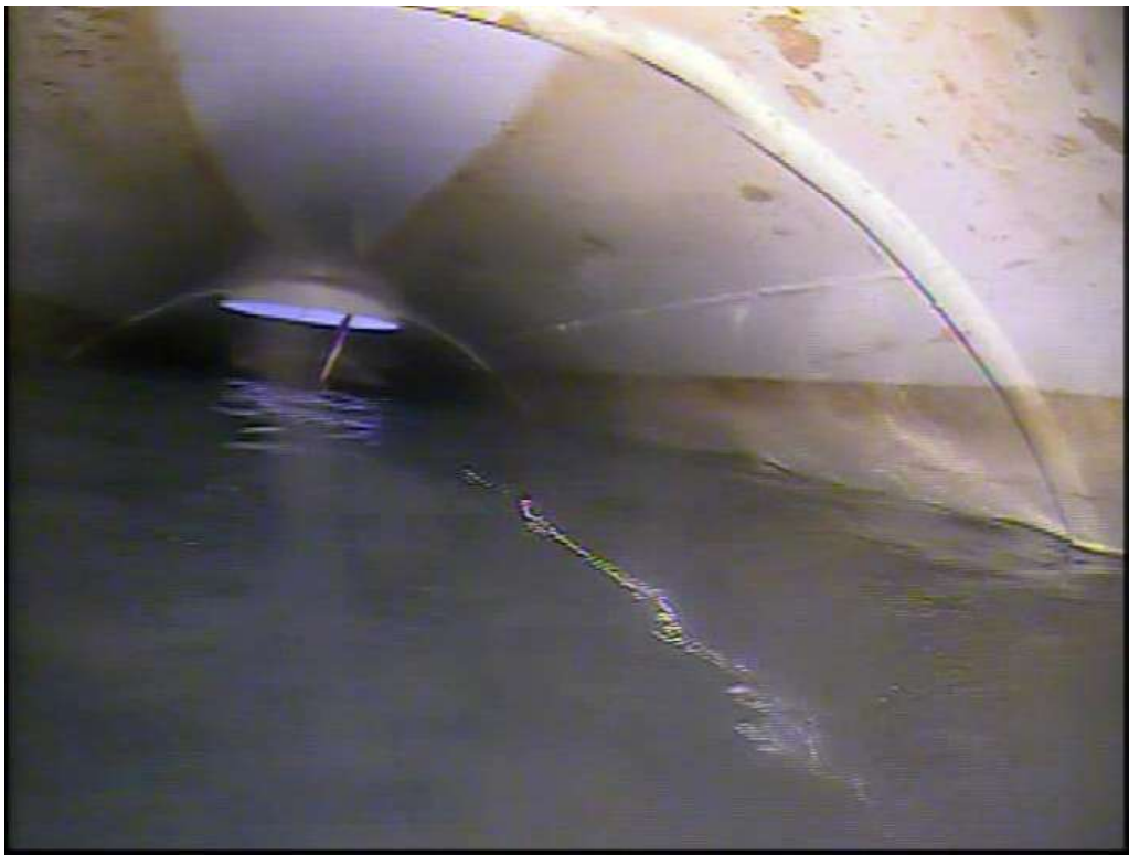
Typical Roof – Staining Noted
